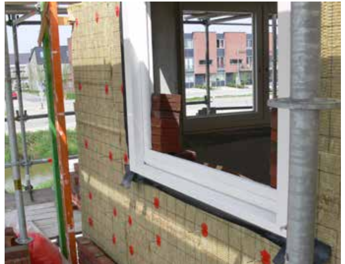
Prikspouwanker met UNI-CLIP
